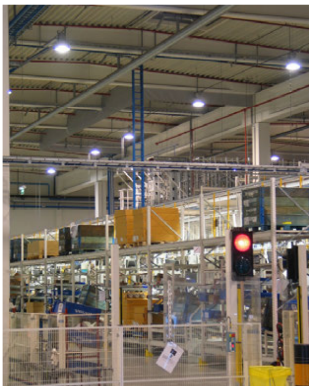
Project draftcurtains - Ghent
